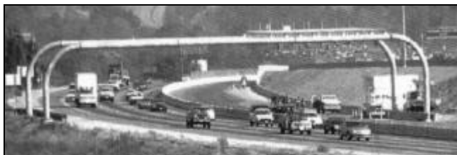
California non-stop toll reader gantry
