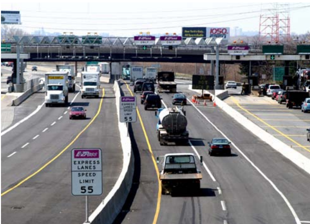
Express E-ZPass traffic is separated from vehicles paying cash well before the toll barrier at NJ Turnpike Exit 18W, reducing weaving and jockeying, promoting safety.
