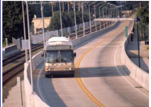
Bus lanes and busways allow buses to escape traffic congestion and provide fast, reliable service. Unlike a train, a BRT bus can effectively serve low-density neighborhoods by leaving the busway. Above, Pittsburgh’s Martin Luther King Busway.
