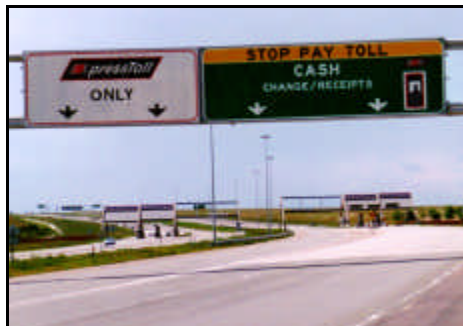
Toll facilities on E-470 in Denver provide a choice between traditional cash toll booths and non-stop, highway speed express lanes for vehicles equipped with an E-ZPass-like electronic tag.
