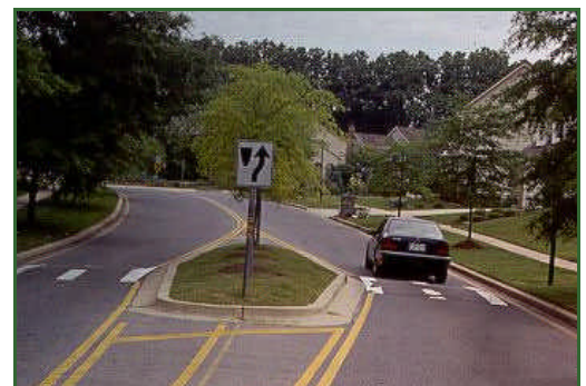
Traffic calming: a median island and speed humps physically slow traffic in a Maryland community.
